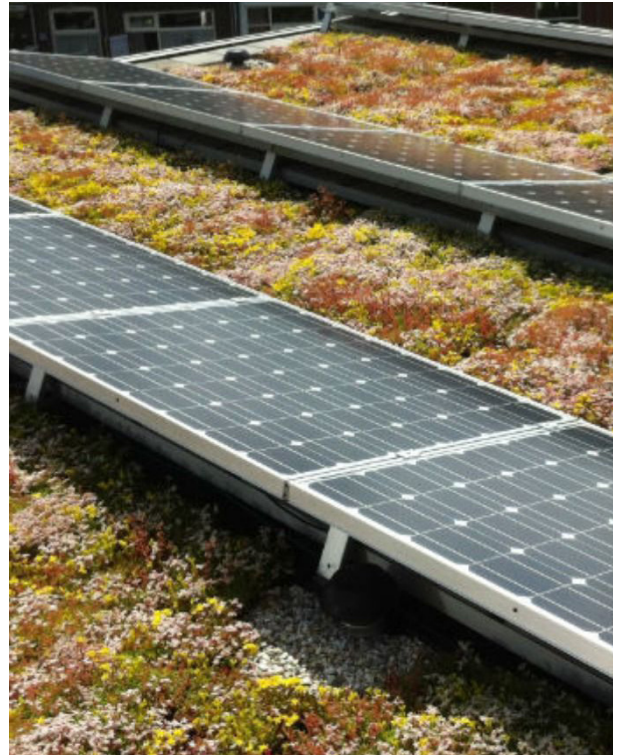
Figure 26 Solar panels on the roof of single storey extensions to the rear of the property are encouraged. This can be in combination with a green roof.
