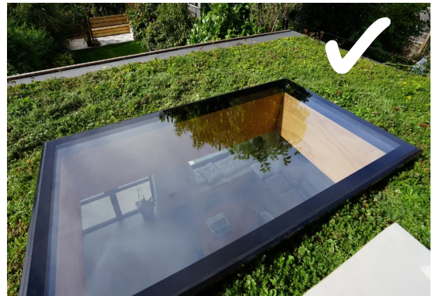
Figure 23 Flat and level sky lights such as this will generally be permitted.
