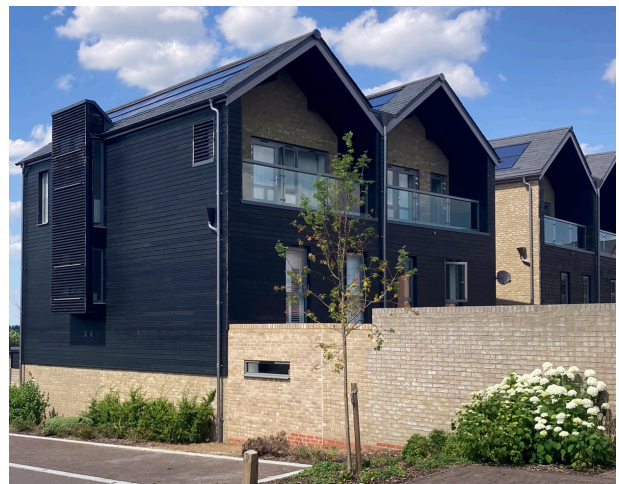
Figure 8 Example where this has been done successfully in Newhall.
