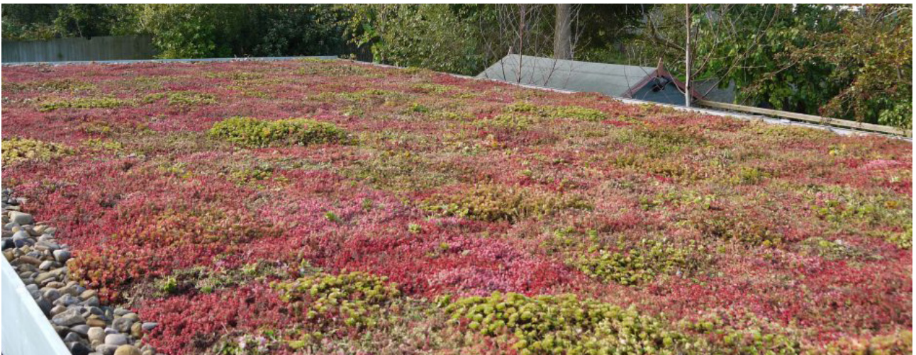
Figure 24 Green roofs provide sustainable drainage, additional insulation and natural habitat. They are also attractive to look down upon from surrounding homes.
