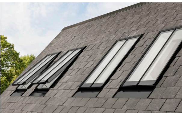
Figure 20 If dormer windows are not acceptable to Newhall Projects, roof windows can provide a possible alternative. Windows with a low profile that lays flush with the roof tiles are preferred.
